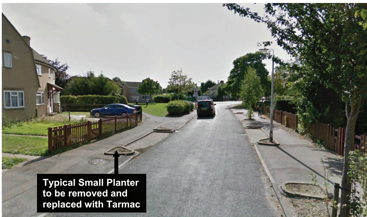
Photo of Existing Location: (View looking towards Water Street)
