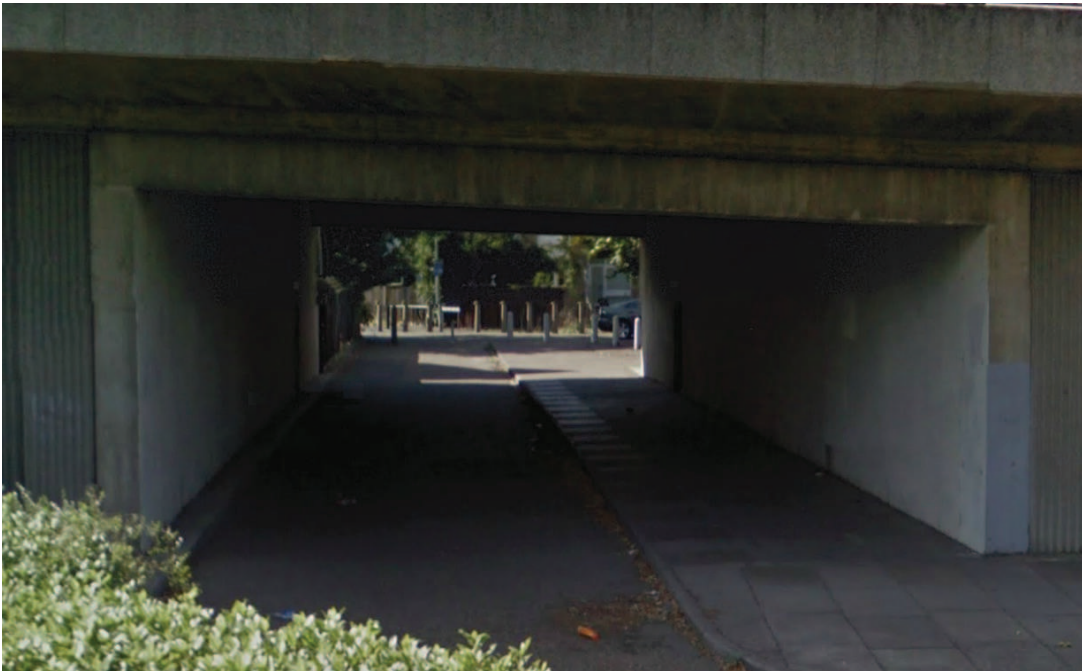
Photo 1 – Existing underpass at Elizabeth Way, looking towards Cutter Ferry Close
